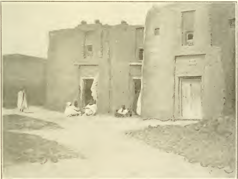
Laing's house, Timboctu.
